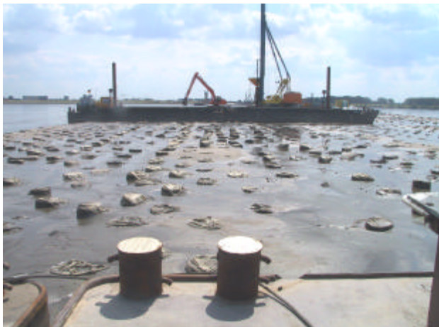
Figure 5. Vibro displacement method from pontoon lying on soft soil.
