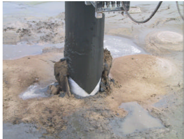
Figure 6. Installed column after drawing the steel pipe under vibration
