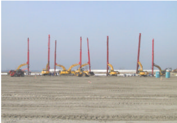
Figure 11. Installation of vertical drains in detail
