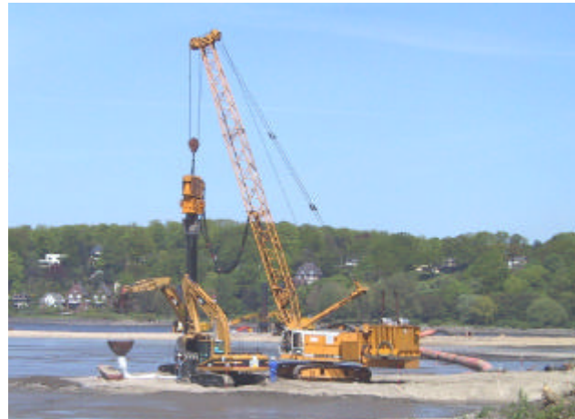
Figure 7. The well-tested vibro displacement method on land.
