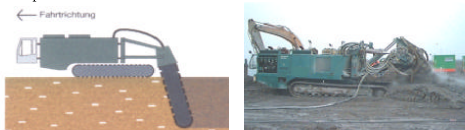
Figure 15. Cut-mix-injection method
