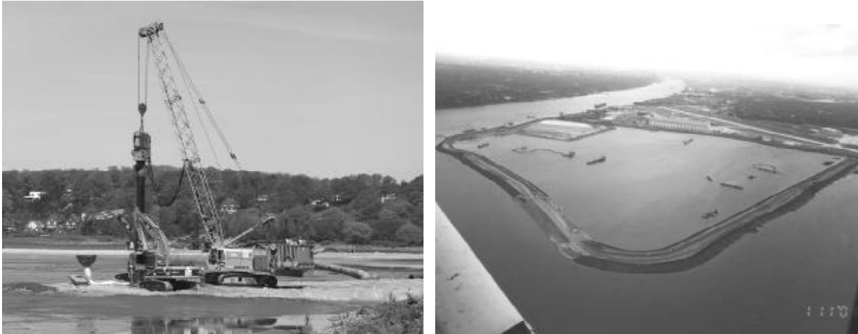
Figure 5 The well-tested vibro displacement method on land and the finished dyke
