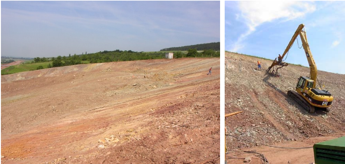
Figure 9. Reconstruction a) flattened slope b) bolting
