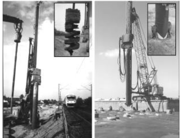
Fig. 2 Excavation and substitution technique with double flap pipe (pictures: Möbius AG)
