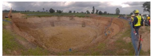
Fig. 2: Building Pit for Shallow Foundation
